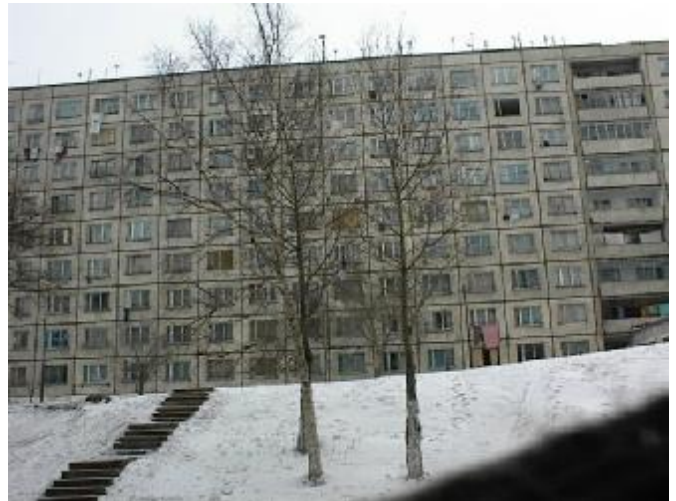
Each window in each dormitory building is a one-room apartment housing a young family. Facilities are down the hall.
