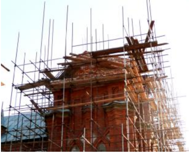
Bricks already rising higher.
