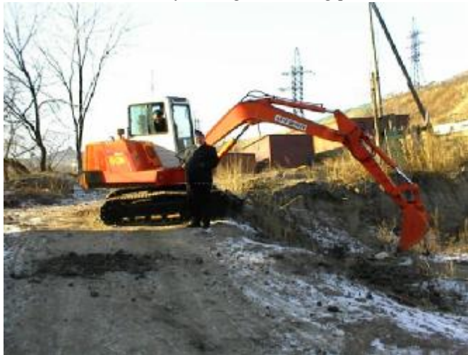
Backhoe starting to work again on the rectory building.
