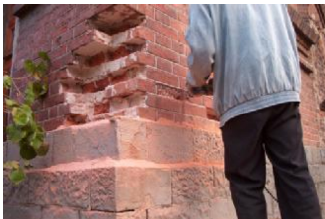
Work on a bad corner.
