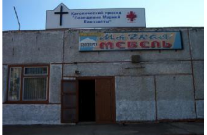
The chapel is at the far end of a complex of furniture stores
