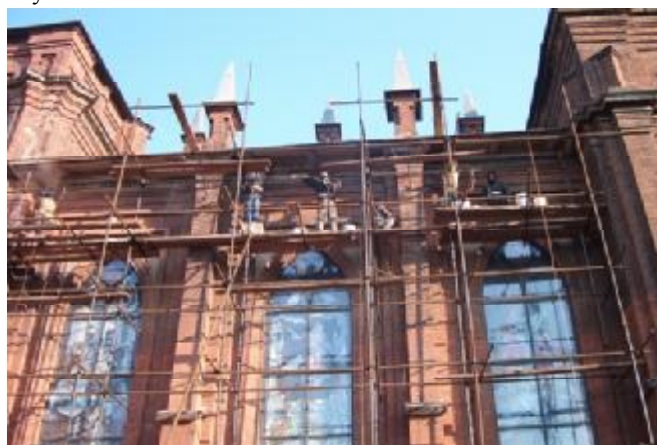
Workers repairing bricks and mortar near the roof.
