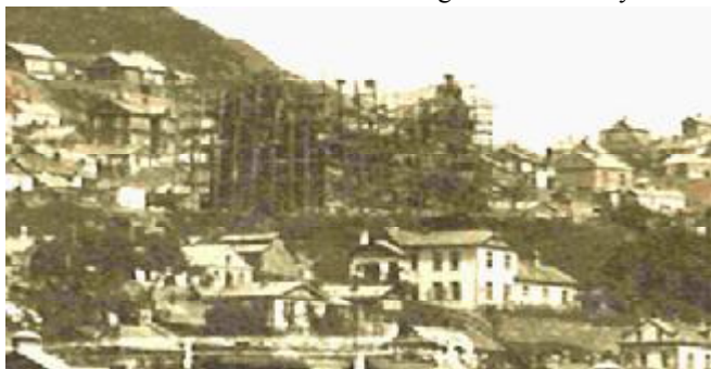
Our church surrounded by scaffold during its construction in 1922.
