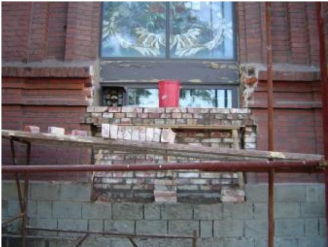
Windows which had been broken into the church walls had to be closed up.
