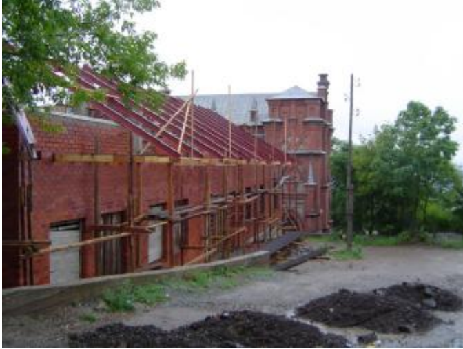
The roof is going up!
