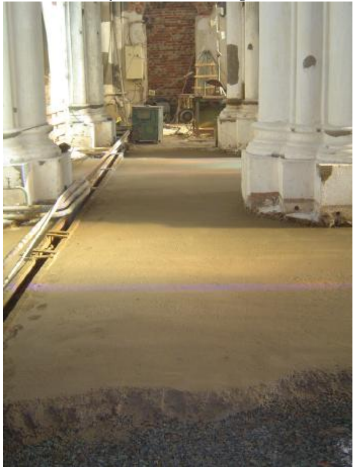
The new concrete floor on which heating coils will be laid.
