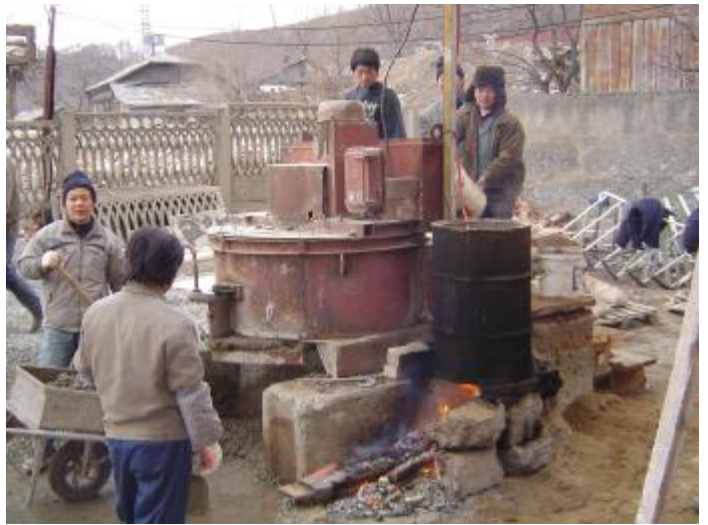
Mixing concrete for the new floor.
