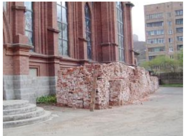
Half the bricks waiting to be used for the steeples.
