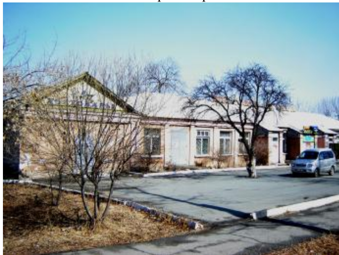
The Romanovka "mall," with the new premises at the left. A mansard roof on a new 2 nd floor, and windows will be added.
