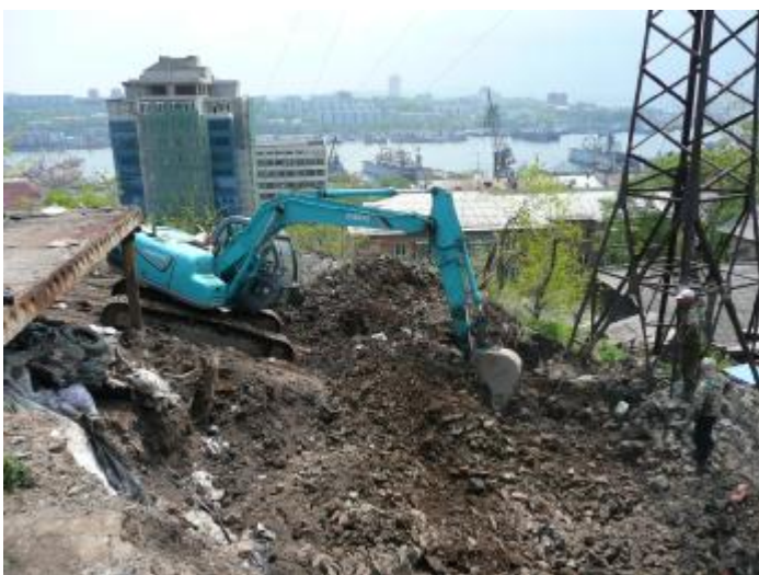
Digging to make way for the new high-tension standards. An old one still stands nearby.
