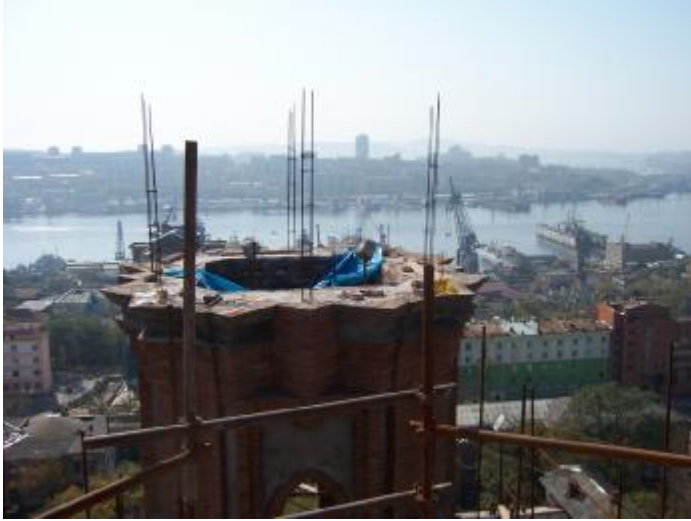
The last layer of brickwork waiting for the metal spire.
