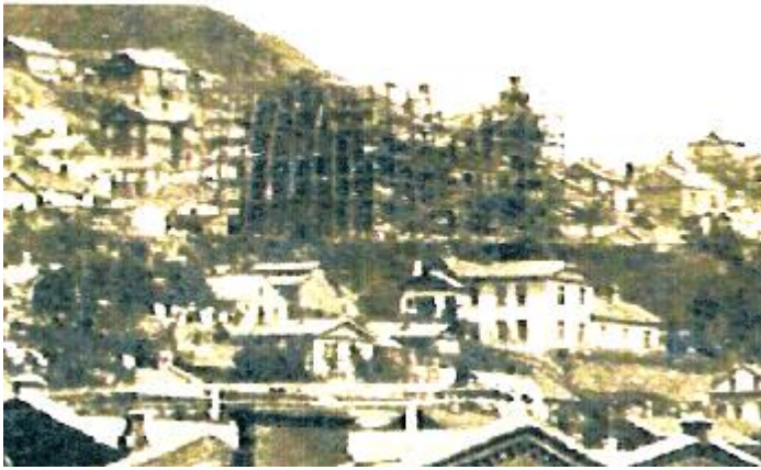
The church surrounded by scaffolds. The only photo we have from the time of the construction of the church, probably from about the time the letter was written.
