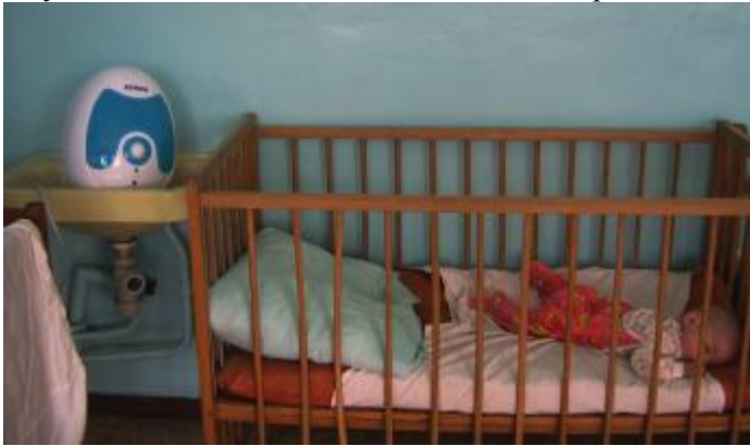
Small water heater looking like a robot peering over a child, is sitting in the sink waiting for installation.
