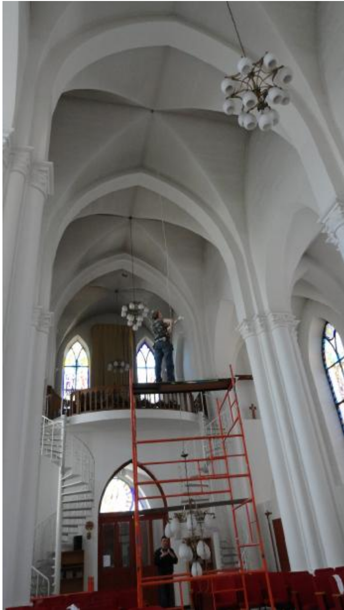
Installing the fire alarm system
