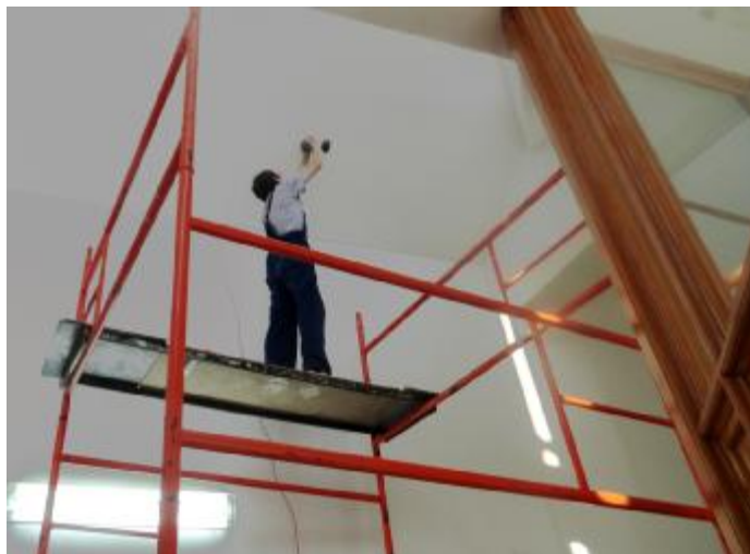
Installing the fire detectors in the monastery
