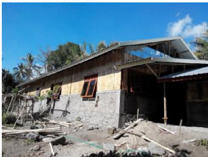
The walls are partially local stones and a metal roof.
