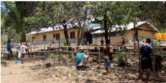
Making a fence around the temporary seminarians' residence building in Maumere
