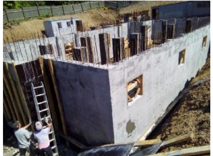
Finishing the basement walls in Nakhodka
