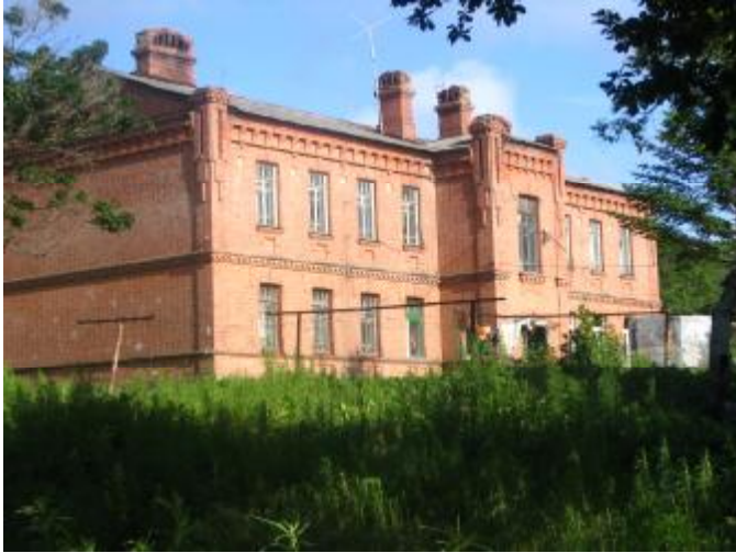
The historic building where the St John's Center will be located
