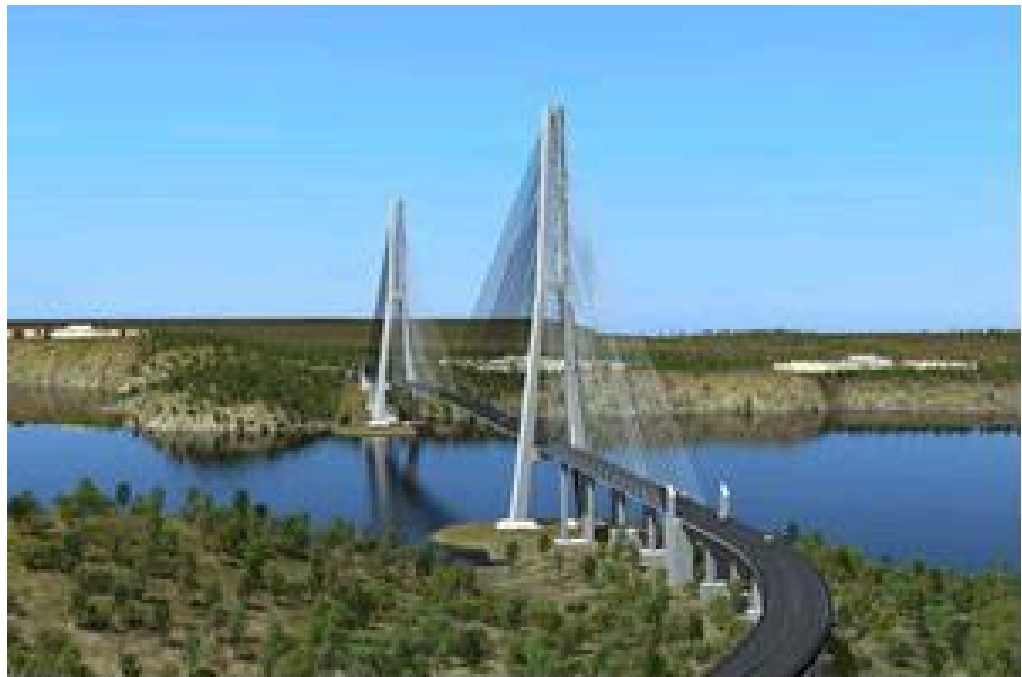
The bridge to Russian Island currently being built.
