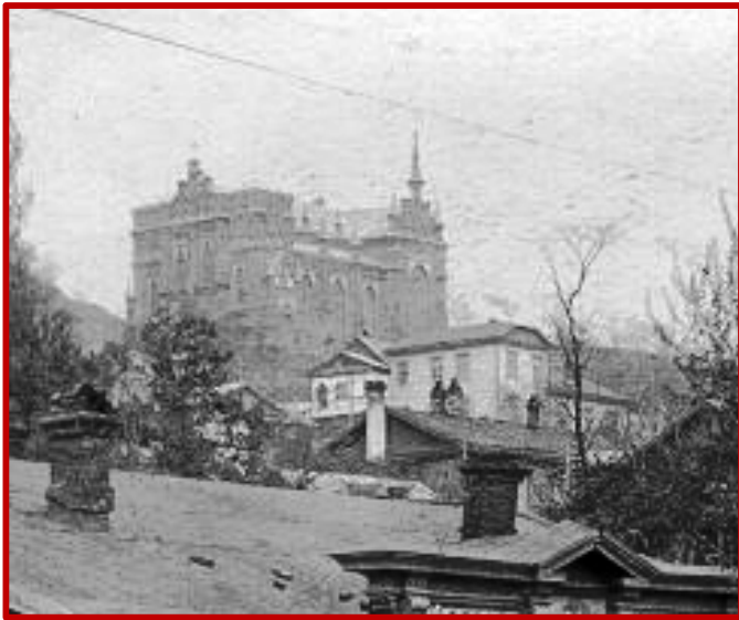
Church nearly done, with small steeples, crosses, but still some scaffolds.
