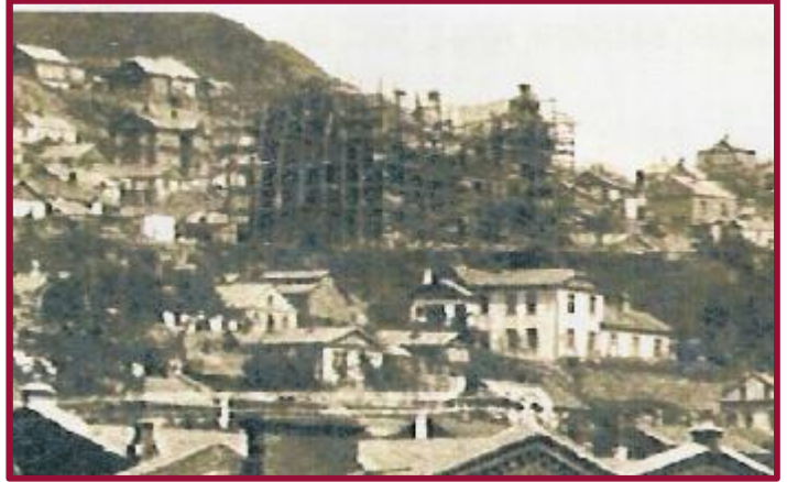
The incomplete church standing in scaffolds
