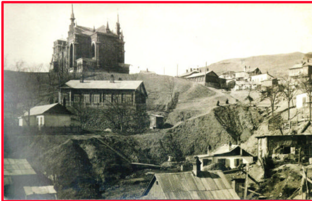
The new church, still without windows, and the old church below it
