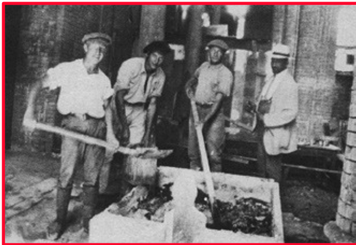
Unidentified German prisoners of war workers who finished the church, with architect Rolf Geyling. Two workers were killed when they fell from the scaffold.
